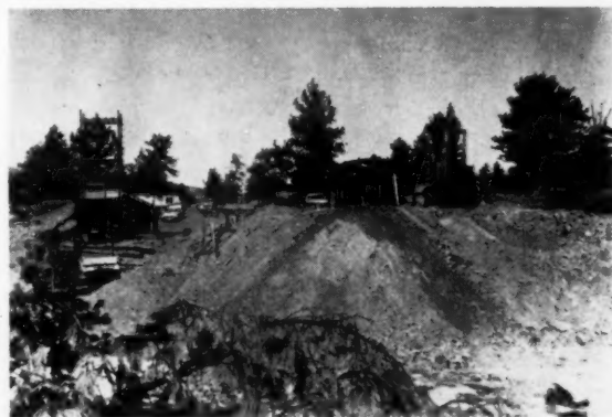
BOOMER MINE with Florman shaft on left and Boomer incline on right. Dump in center assays about 3.0 percent BeO.
